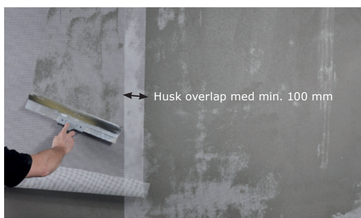
Overlap med minimum 100 mm
