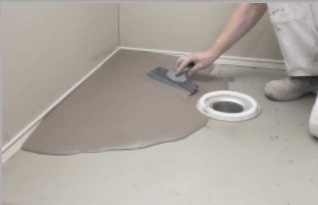
Building drainage slope
