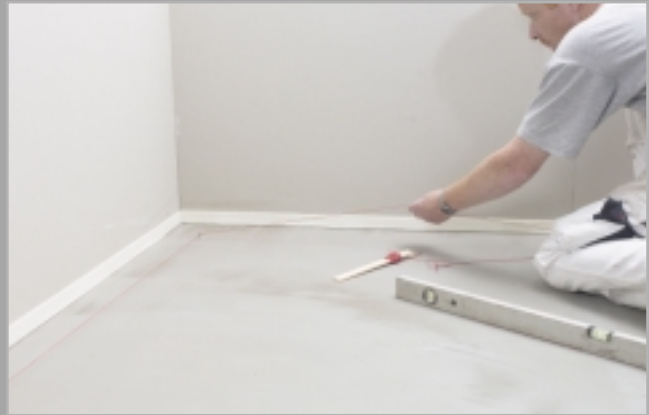
Tightening the line
