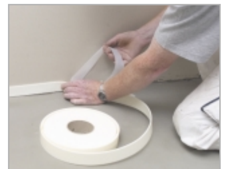
Foam tape: Application on wall
