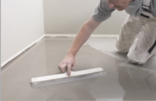
Spreading with trowel
