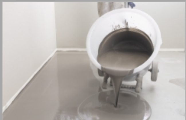
Pouring the levelling compound
