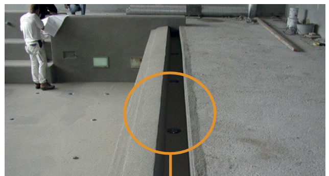
Fitting of Alfix VT sealing strip
