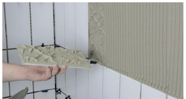
Checking the adhesive coverage
