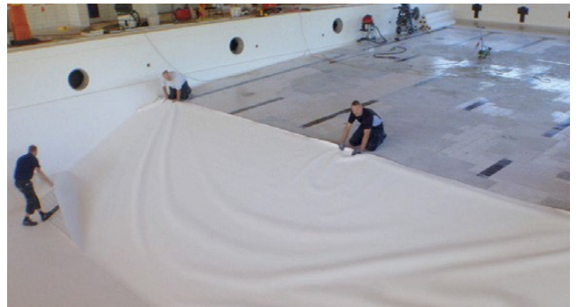
Fitting PVC liner
