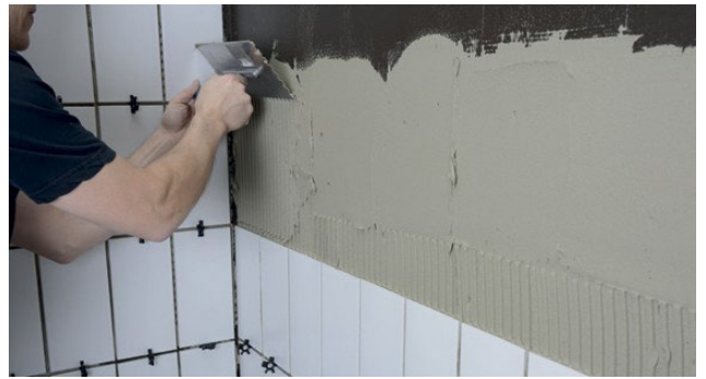
Applying tile adhesive using a notched trowel
