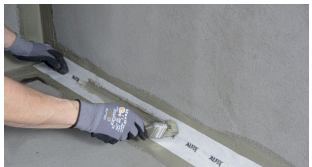
Fitting of Alfix VT sealing strip
