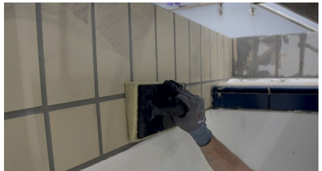
Wash the joints using a well-wrung viscose sponge.
