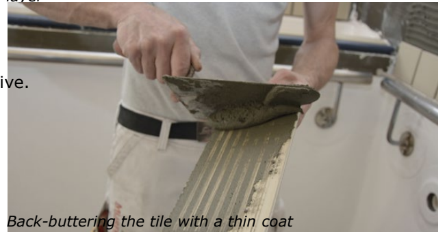
Applying the contact layer
