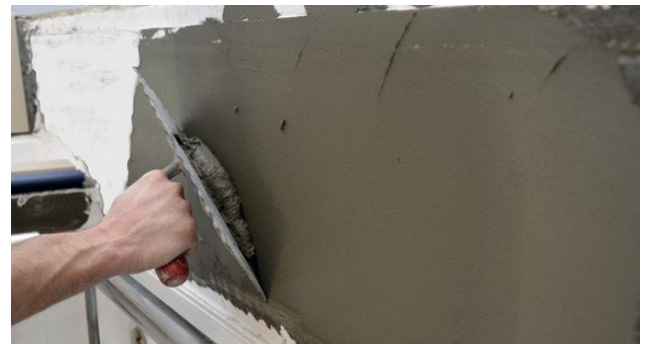
Applying the contact layer
