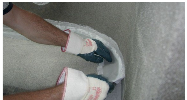
Fitting of Alfix VT sealing strip
