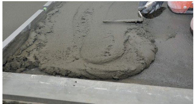
Applying and compressing the layer on the floor
