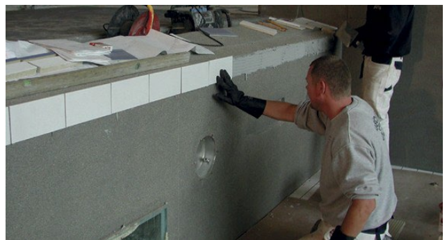
Fitting tiles onto the wet adhesive.
