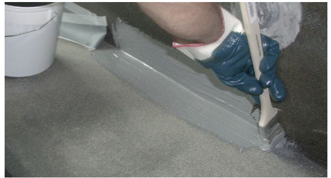
Application of Alfix Epoxy Membrane
