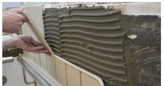
Fitting the tiles
