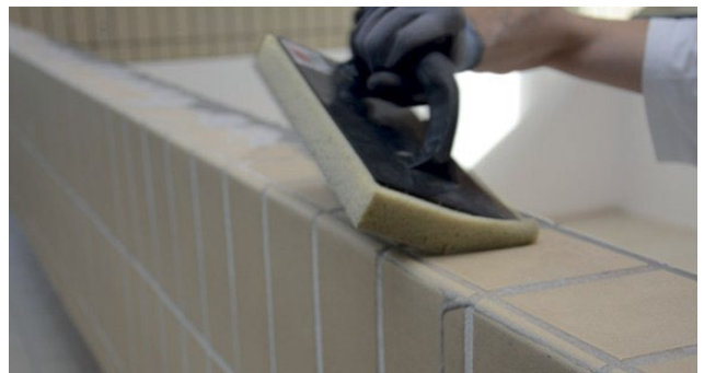
Adjust the joints to match the tile design
