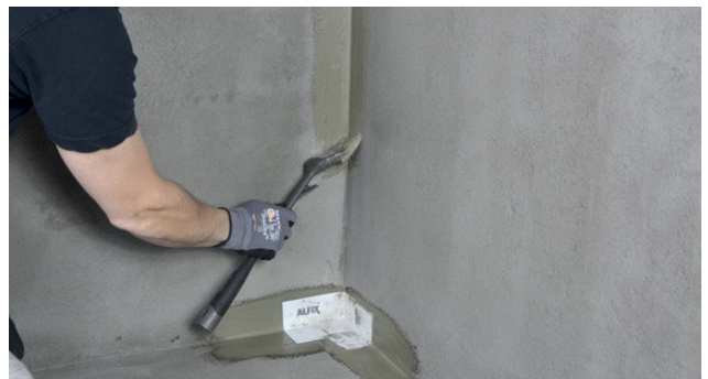
Fitting of Alfix VT corner in the sealing membrane.
