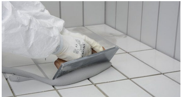
Applying on floor using an epoxy grout float
