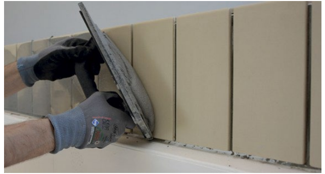
Applying Alfix IndustryFuge - CeraFill 18
