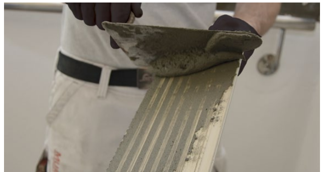
Back-buttering the tile with a thin coat
