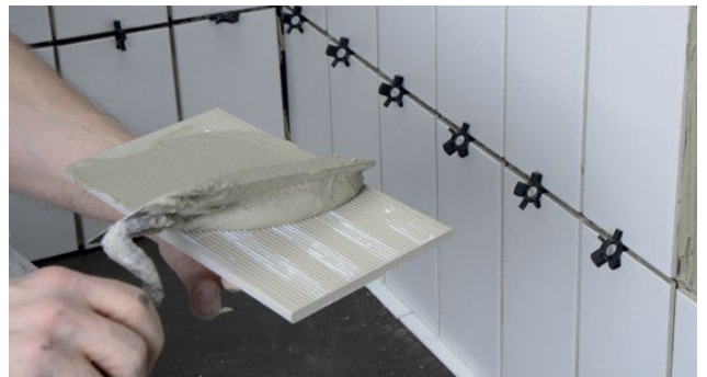
Back-buttering the tile with a thin coat
