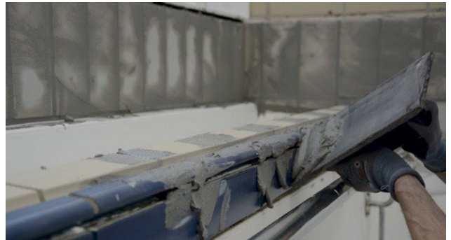
Joints must be filled completely
