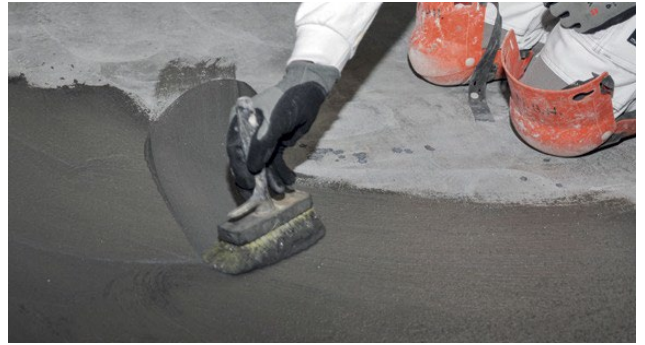
Slurry bonding
