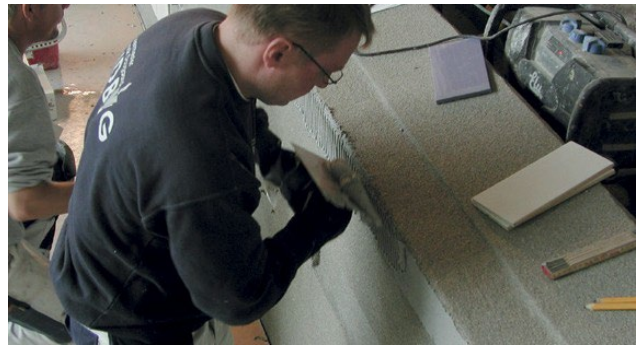
Applying Alfix C2 Epoxy using a notched trowel
