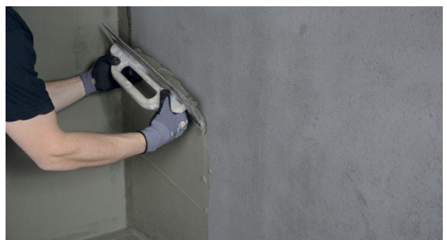
Applying Alfix 2K Sealing Membrane – pore filling coat
