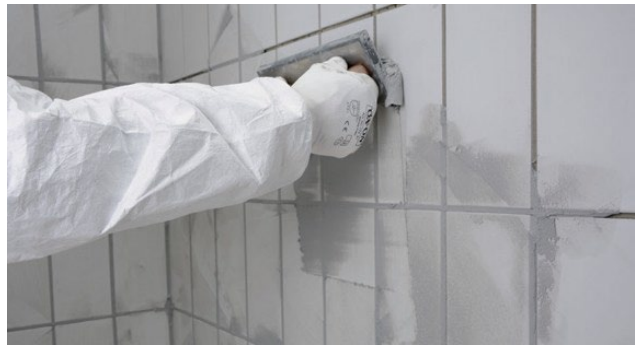
Applying on wall using an epoxy grout float
