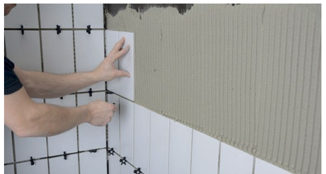
Fitting the tiles
