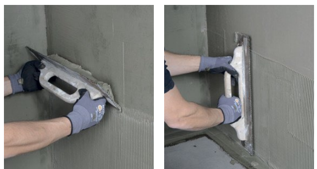
Applying 2K Sealing Membrane and smoothing
