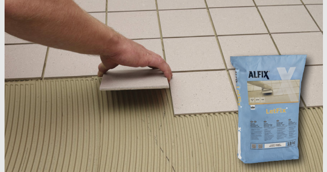
Flismontering i Alfix flislim
