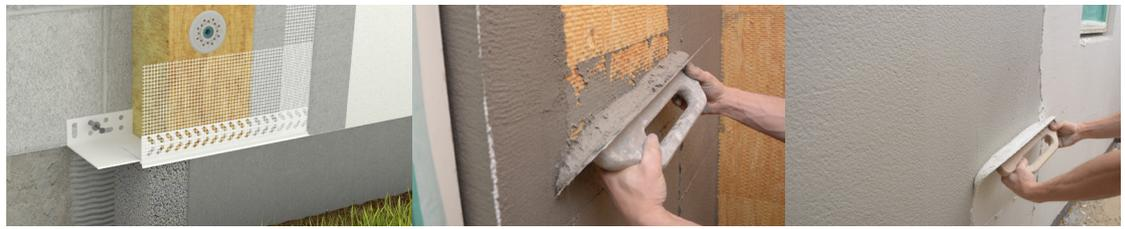
**Duratherm complete:** A complete thermal insulation system consisting of the correct amounts of insulation boards, facade adhesive, bonding and thin coat render as well as accessories for reinforcement of external render. The brick layer is now free to focus on his primary job, rendering.
