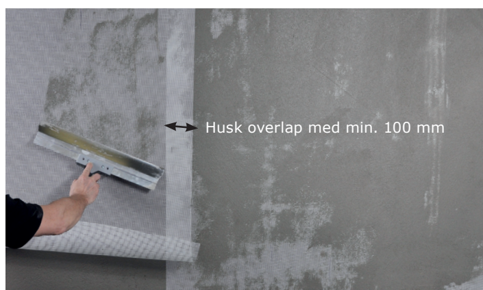
Overlap med minimum 100 mm
