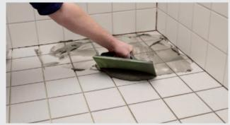
Grouting with cement-based grout
