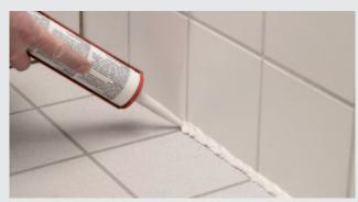
Sealing with silicon sealant
