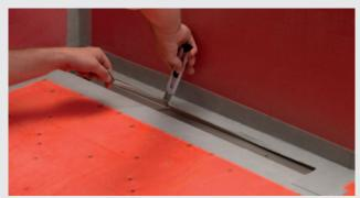
Trimming edges around linear channel drain
