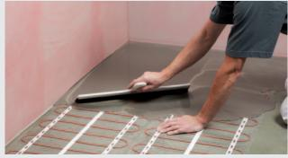
Application and spreading of levelling compound
