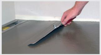
Producing slope towards linear channel drain
