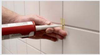
Filling hole with silicone sealant
