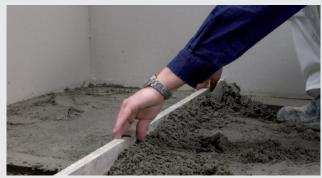
Screeding onto timber joist system
