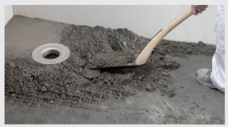
Producing slope with screeding mortar
