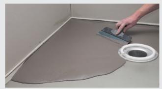
Producing slope around conventional floor drain
