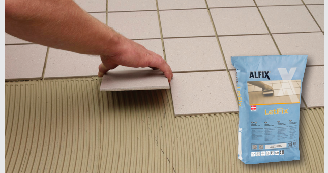
Flismontering i Alfix flislim
