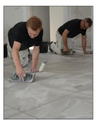
The grout is suitable for ceramic and quarry tiles and mosaics with moderate or low suction.
